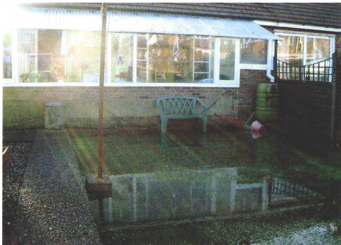
No 2 Brooklands Road – Regular occurrence, raw sewage in garden. No 4 Brooklands Road has a back-flow and cannot use the toilet on these occasions.
