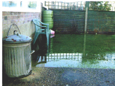
No 2 Brooklands Road – Regular occurrence with raw sewage in garden.
